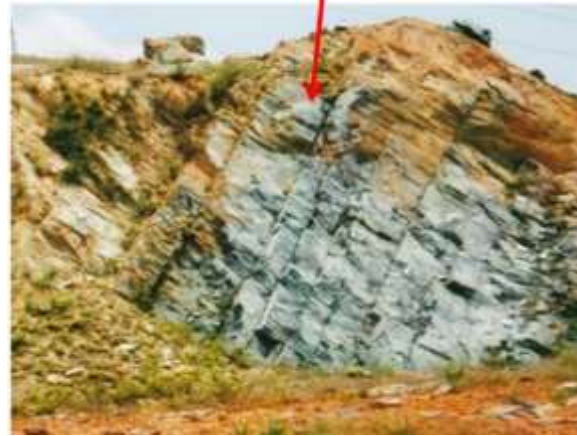
Fig. 1. Granite cut slope in Kajang SILK Highway at location 2.961250°N, 101.719436°E
