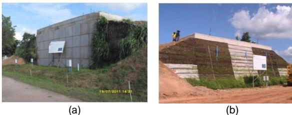
Figure 7. Photographs of test embankments: (a) vertical face with metallic reinforcements and (b) sloping face with polymer reinforcements.
