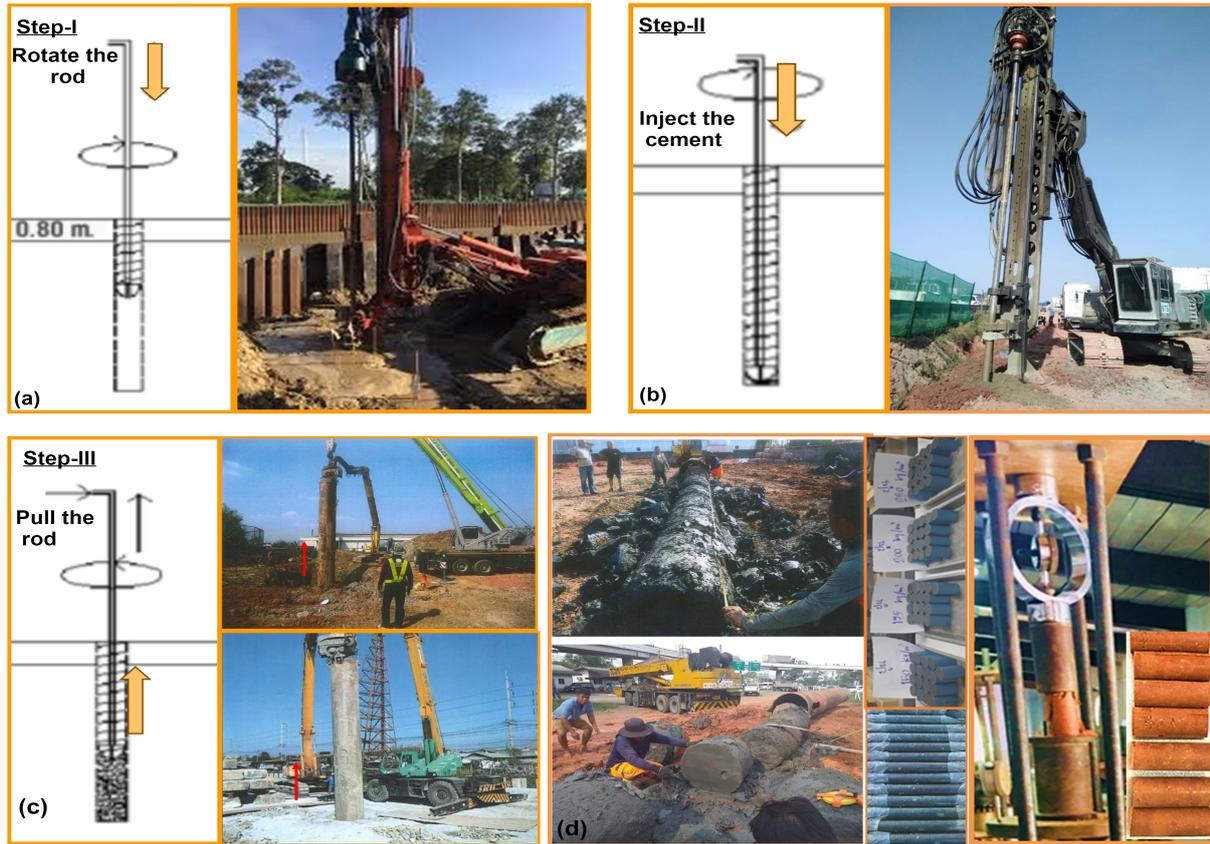
Fig. 1. Sketch and corresponding photographs from (a) to (c) describe the methods of dry process, cement inject and pull out of soil-cement column by means of pull out test and, (d) represents the preparations of cores extracted from the pull out test and laboratory undrained strength tests.
