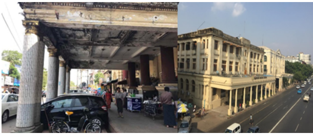
Fig.7 Building with Big canopy along main road
