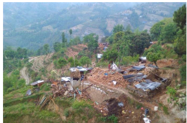
Fig. 4. Collapse of residential buildings in Nayagaun settlement (Source: Santosh Lama, ward 3 beneficiary)
