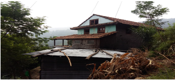
Fig. 11. House in Nayagaun that survived after Gorkha Earthquake
