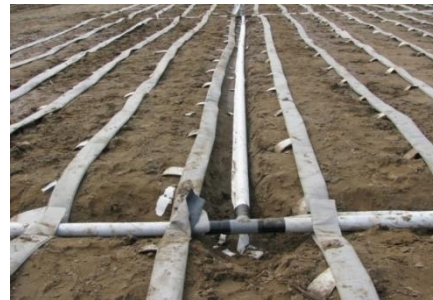
Fig. 9. VCM-MB using airtight membrane and horizontal.
