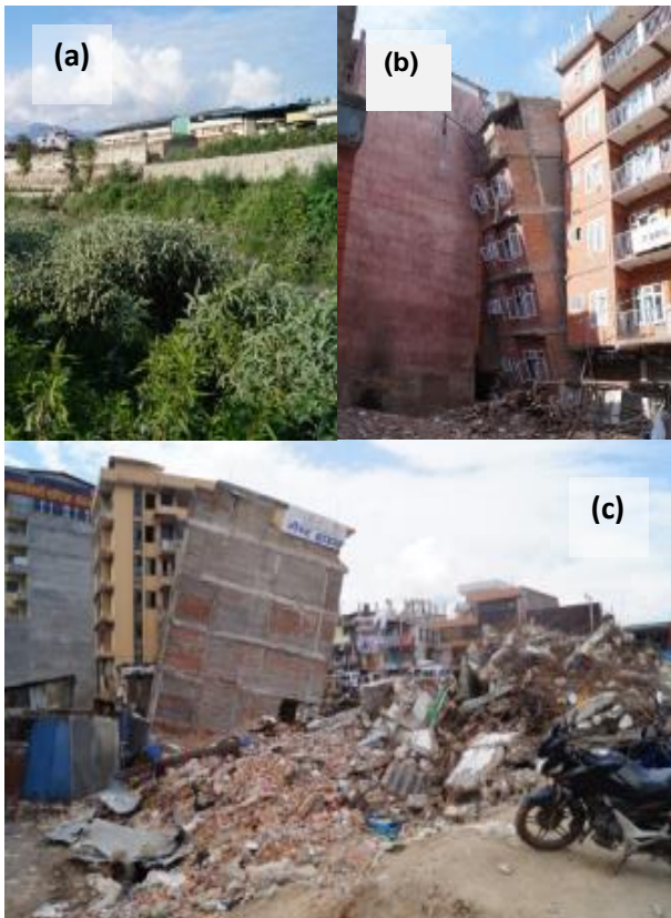
Fig. 3 (a). Photo adjacent to river and flood plain deposits showing building built on soft lake deposits with Kathmandu with (b) and (c) examples of collapsed buildings within Kathmandu in vicinity to Fig. 3 (a), showing the potential impact of building on superficial deposits
