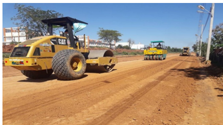
Fig. 1. The Road Construction with Loess
