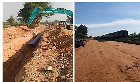
Fig. 2. The Infrastructure and Pavement and Railway Construction with Loess
