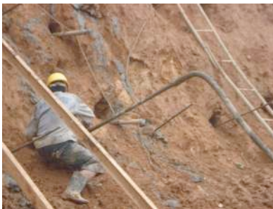
Fig.14c. Inject cement grout
