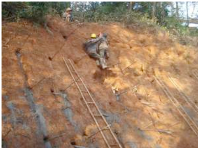
Fig.14b. Install rebar steel d=18mm
