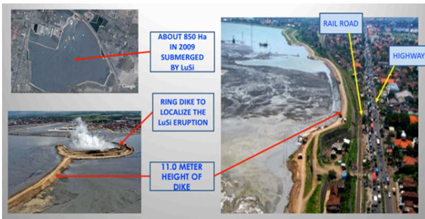
Fig. 2. Dike built surrounded the Lumpur Sidoarjo (LuSi) area
