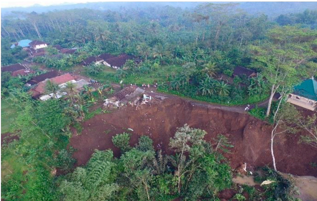
Fig. 1. Slope failure occurred in Sumberjo Village, Blitar Indonesia (Alexander, 2017).
