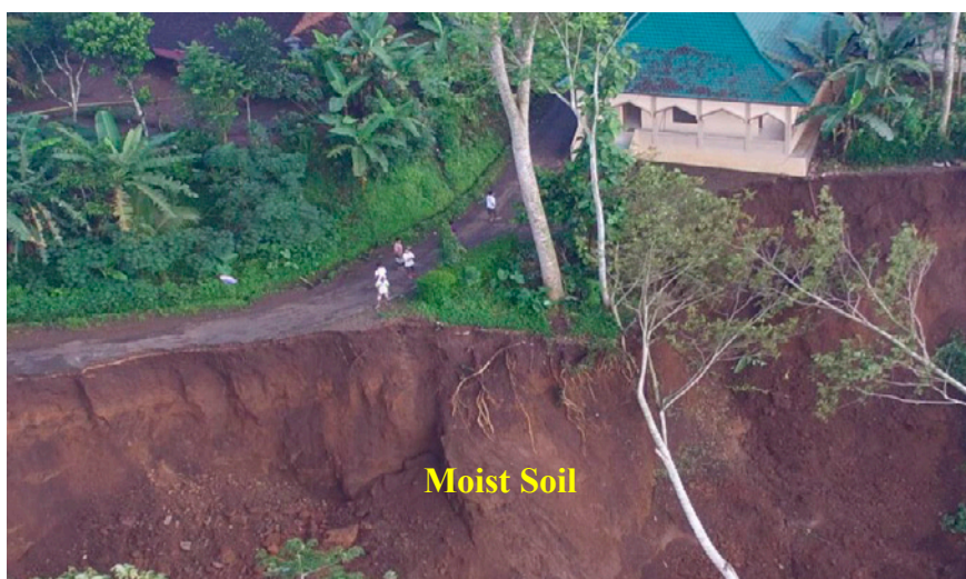
Fig. 2. Typical mostly dry and moist soil layers along the failed slope (assumption of saturated slope prior to failure is not proven). (Source: Alexander, 2017).
