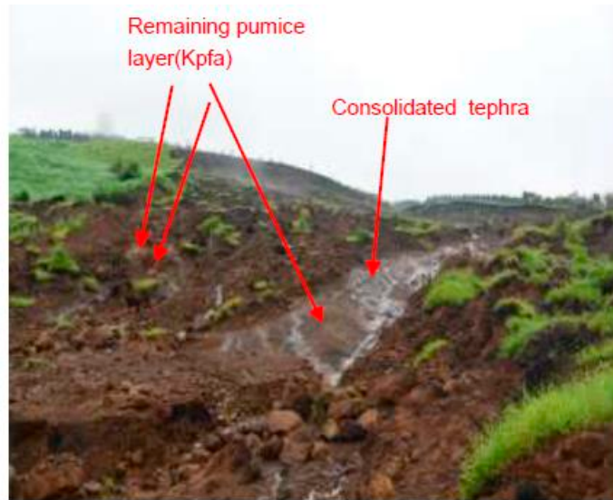
Photograph 2 : Landslide that occurred on a slope of the Takanoobane lava dome.
