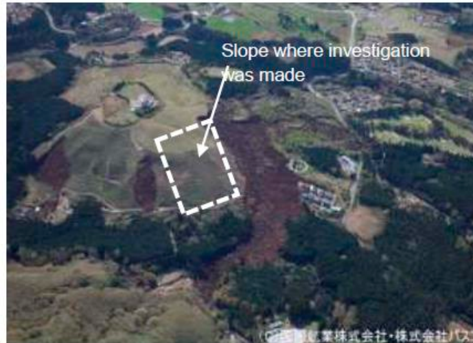
Photograph 1 : Landslide that occurred on a slope of the Takanoobane lava dome.
