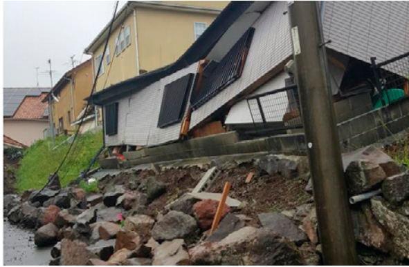
Fig. 1. Houses damages due to subsidence.
