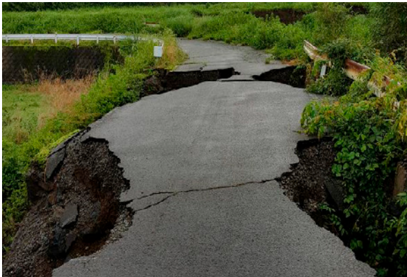
Fig. 3. Damages to road.
