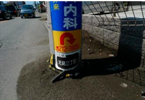
**Fig. 9.** An electric pole settled by more than 1 meter (Chikami, Minami-ku, Kumamoto City, 32.765147N, 130.687960E)
