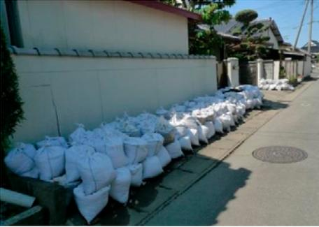
**Fig. 7.** Sandbags refilled with 25 kg sand boil deposits removed from a 4 meter-deep well. The number of sandbags reached 320 in total (8 ton in weight) (Chikami, Minami-ku, Kumamoto City, 32.769953N, 130.691958E)
