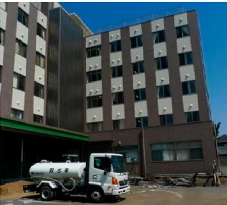
**Fig. 8.** A five-story building constructed three years ago lifted because of a 1-m ground subsidence (Chikami, Minami-ku, Kumamoto City, 32.769215N, 130.691603E)
