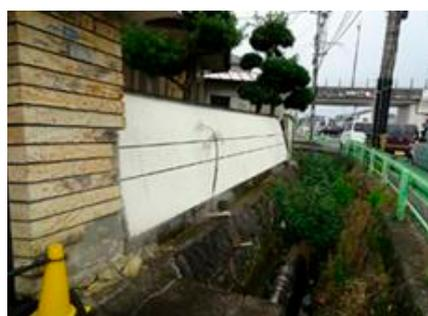
**Fig. 6.** Tilted wall due to liquefaction (Chikami, Minami-ku, Kumamoto City, 32.770945N, 130.692849E)
