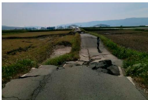
**Fig. 16.** Two-meters of settlement and lateral displacement of a farm road. Length of the settlement was approximately 50 m (Yakuinbaru, Aso City, 32.949986N, 131.084916E).
