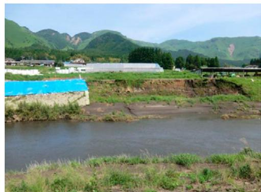
**Fig. 14.** Collapsed levee of the Kurokawa river and sand boils at the foot of the levee (Akamizu, Aso City, 32.926322N, 130.991291E)
