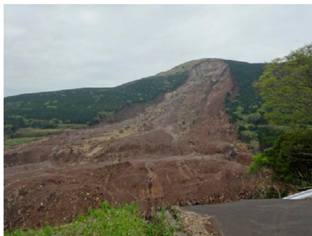
Fig. 2. Image overview of large-scale slope failure covering the Aso-ohashi Bridge.
