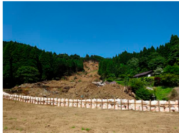
Fig. 8. Image showing an overview of surface failure.
