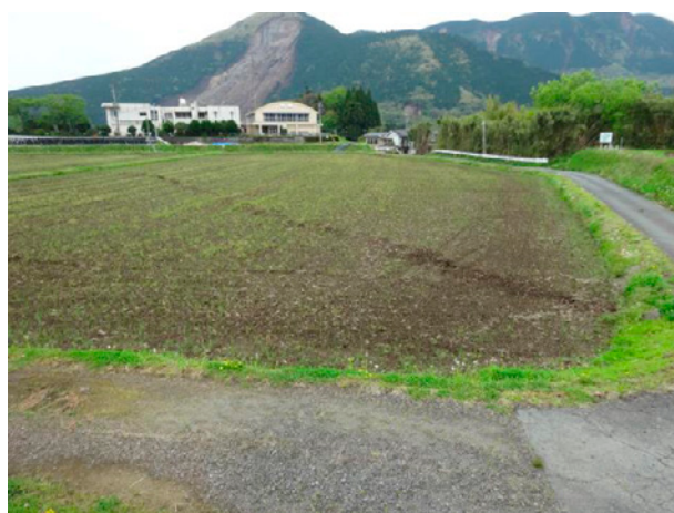
Fig. 4. Image showing surface cracks exposed on the opposite side of the large-scale slope failure.
