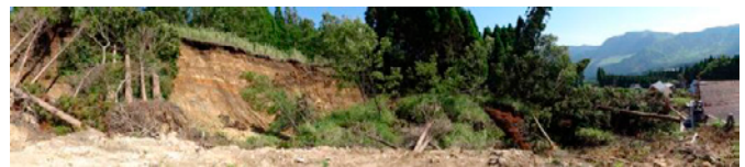
Fig. 9. Image showing an overview of another surface failure.
