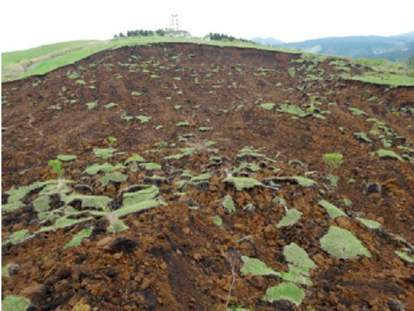
Fig. 5. Image of the landslide at Takanodai.
