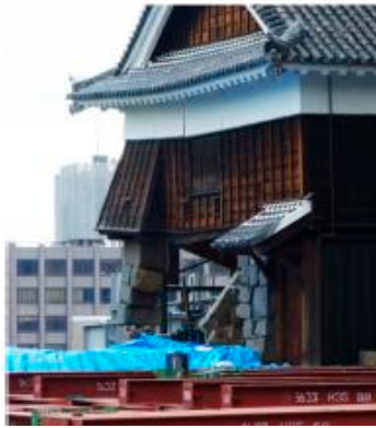
Fig. 6. Photograph of the stone wall of lidamaru Yagura (2004 reconstruction), which was constructed using the Sangi-tsumi method. (courtesy of Prof. K. Meguro, taken Oct. 26, 2016)
