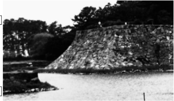
Fig. 2. Photograph of the shallow slope of a stone wall at Hagi Castle, Yamaguchi Prefecture, Japan (photo by T. Ohsumi, taken in 1990).
