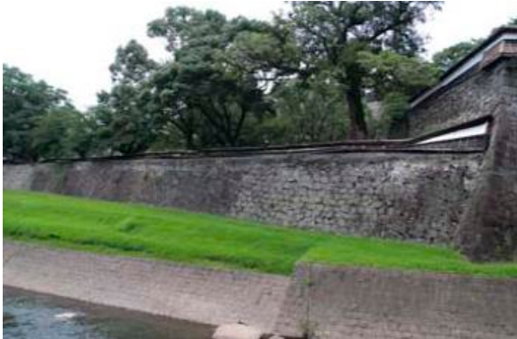
Fig. 27. Photograph of the longest wall in the castle, Naga-kabe, along Tsuboigawa river. An 80-m-long section of this wall collapsed after the earthquakes (photo by T. Ohsumi, taken July 20, 2016)
