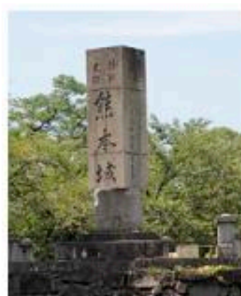
Fig. 31. Photograph showing stone monument rotated by the main shock (photo by T. Ohsumi, taken July 20, 2016)
