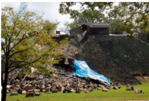
Fig. 24. Photograph of Kita Juhachiken Yagura . Located between Kato Shrine and Kumamoto Daijingu shrine, this turret completely collapsed (photo by T. Ohsumi, taken August 11, 2016)
