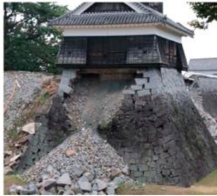
Fig. 7. Photograph of the stone wall of Inui Yagura (2003 reconstruction), constructed using the Sangi-tsumi method. (photo by T. Ohsumi, taken Aug. 11, 2016)
