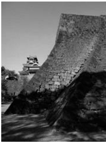
Fig. 3. Photograph of the Niyo stone walls of the Kumamoto Castle. Kato family age (shallow slope: front part). Hosokawa family age (steep slope: inner part)(photo by T. Ohsumi, taken in 1989).
