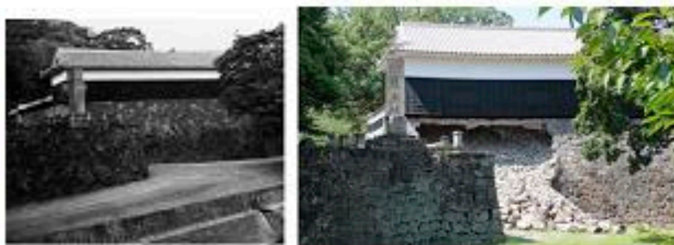
Fig. 29. Photograph of Bagu Yagura-dai before (left; photo by T. Ohsumi, taken in 1989) and after the earthquakes (right; photo by T. Ohsumi, taken August 11, 2016)
