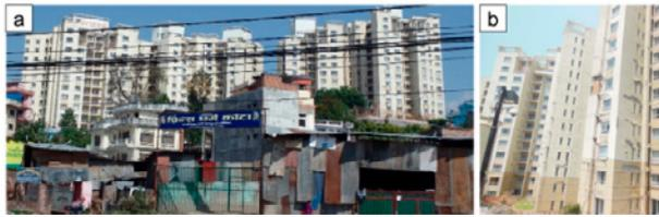
**Fig. 11.** (a) Park View Horizon apartment (N: 27.739762°, E: 85.324410°) was severely devastated by the main shock due to the basin effect, and (b) close view.
