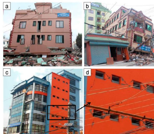
Fig. 8. Damaged buildings at (a) Gongabu (N: 27.738114°, E: 85.307635°), (b) Machhapokhari (N: 27.735511°, E: 85.305340°), (c) Newly constructed building at Tripureshwar, Kathmandu along the Tukucha River and (d) severe diagonal cracks on the wall (N: 27.691972°, 85.316163°).
