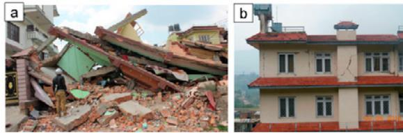
**Fig. 10.** Performance of a RC building on new fill at (a) Purano Naikap (N: 27.700051°, E: 85.264569°), Kathmandu and (b) Balaju (N: 27.742651°, E: 85.300751°).
