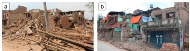
**Fig. 15.** Almost completely destroyed old town at (a) Madhyapur Thimi, Bhaktapur (N: 27.678854°, E: 85.404766°) and (b) Balaju, Kathmandu (N: 27.736054°, E: 85.302531°).
