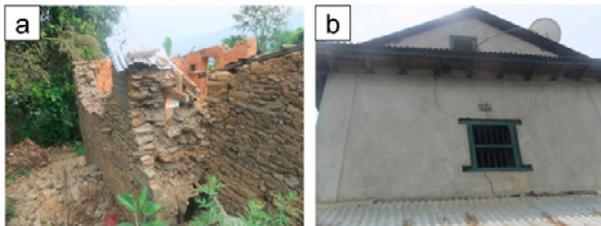
**Fig. 21.** (a) Stone masonry building, a residential house collapsed on the ridge line and (b) cracks on the wall of the building located on the ridge line.
