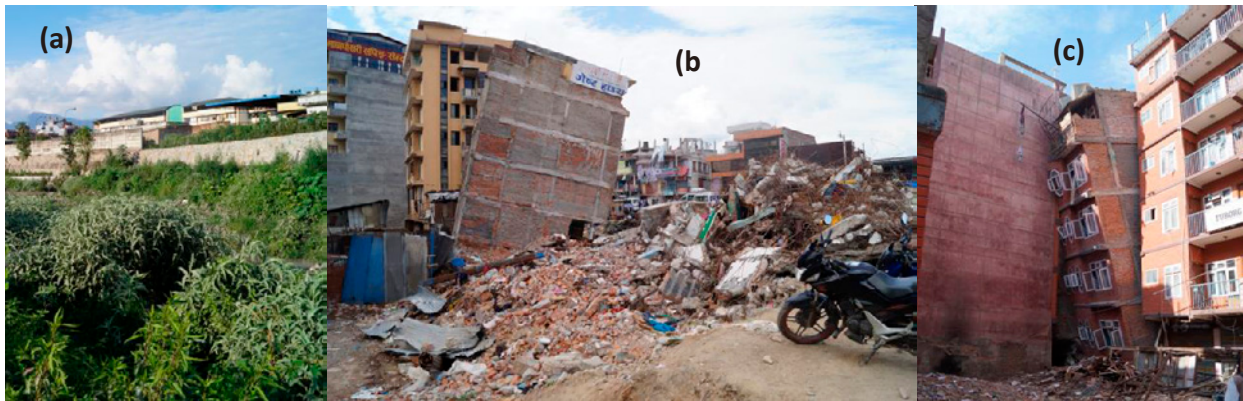
Fig. 13. (a) Building on soft lake deposits with Kathmandu (b) and (c) examples of collapsed buildings within Kathmandu in vicinity to Fig. 13(a).
