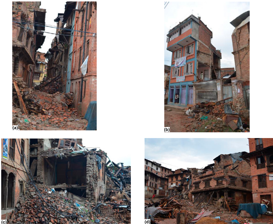
Fig. 7. Damages around Naag Pokhari and Khala of Bhaktapur Durbar square. Many old-aged buildings were severely damaged together with occasional new buildings due to inadequate construction.
