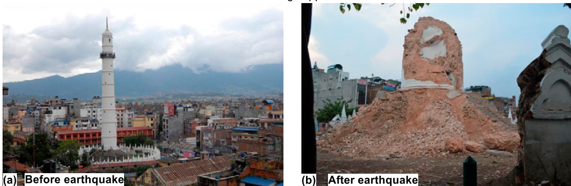
Fig. 16. Bhimsen Tower also called Dharahara (a) before the quake (Courtesy: http://www.nytimes.com/ ) and (b) collapsed after the quake.
