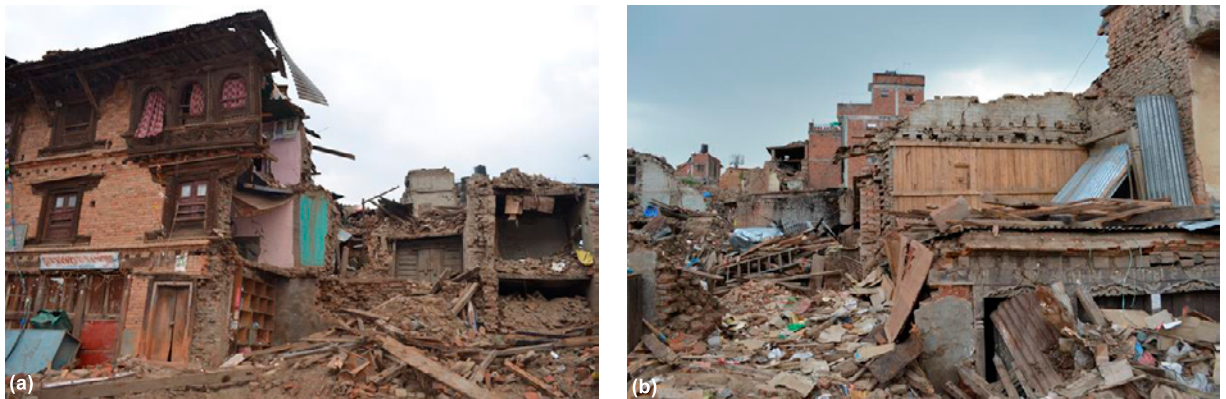
Fig. 4. Damages on ancient Newar town of Sankhu area.
