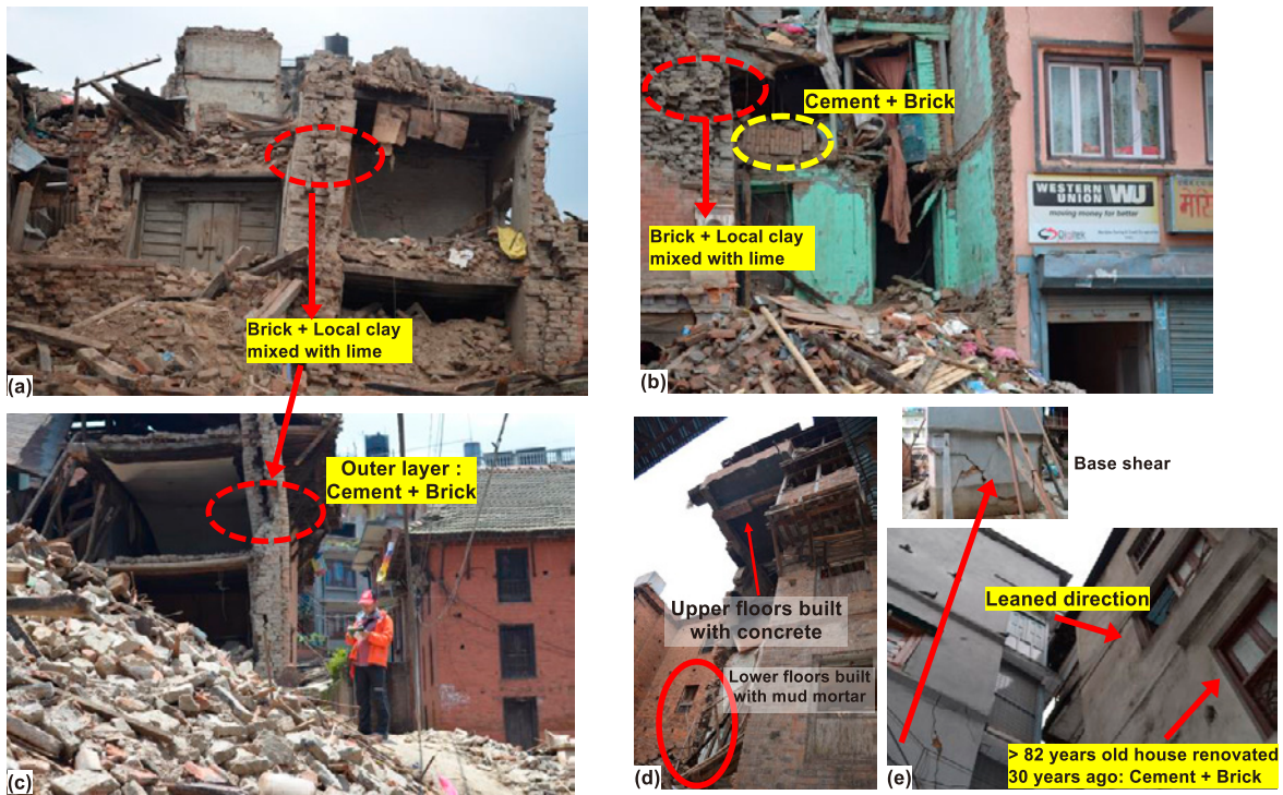
Fig. 36. Figures from (a to d) represent non-engineered practices of renovation and (e) left house renovated one year before the quake without considering engineering design, as a result base shear formed and leaned towards next house. Meanwhile, the right side of the house was also renovated 30 years ago with completely replaced mud + brick with cement + brick and withstood the main shock and aftershock with only minor cracks inside the house. This house is older than 82 year and existed during the 1934 EQ.
