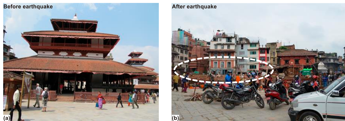
Fig. 9. Photograph representing Kasthamandap (Maru Satath): (a) Before earthquake (Courtesy: Wikipedia) and (b) After the earthquake. The name of the Capital Kathmandu is originated from this historical shrine.
