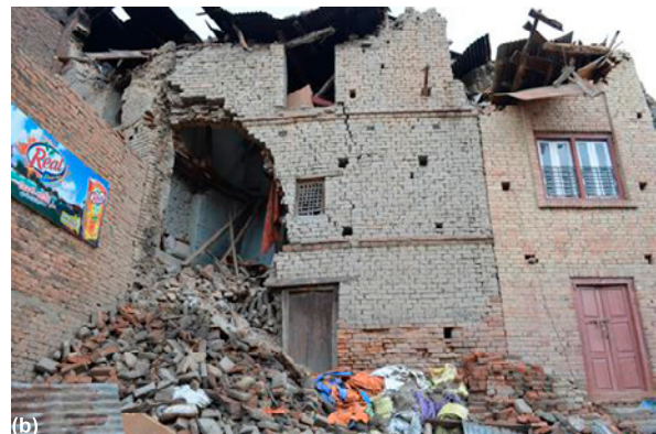
Fig. 2. April 25 main shock and May 12, 2015 aftershock contributed to intensive damages on old aged buildings. Photograph represents areas from (a) Bhatkapur and (b) Sankhu.
