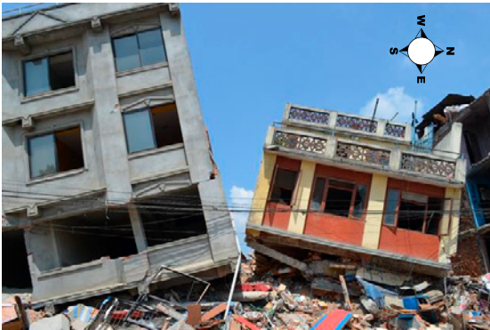
Fig. 22. Tilted RCC building near Sitapaila, Ringroad, Kathmandu. Tilted towards N-S directions.
