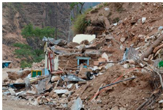
Fig. 27. Houses were at the toe of the slope was demolished completely by earthquake induced landslides along the Araniko Highway.
