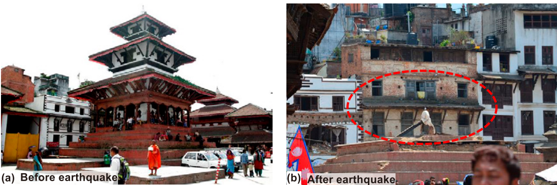
Fig. 12. Trailokya Narayan Mohan temple (a) before the quake (Courtesy: http://hanumandhoka.gov.np/ ) and (b) collapsed all three-stories after the quake.
