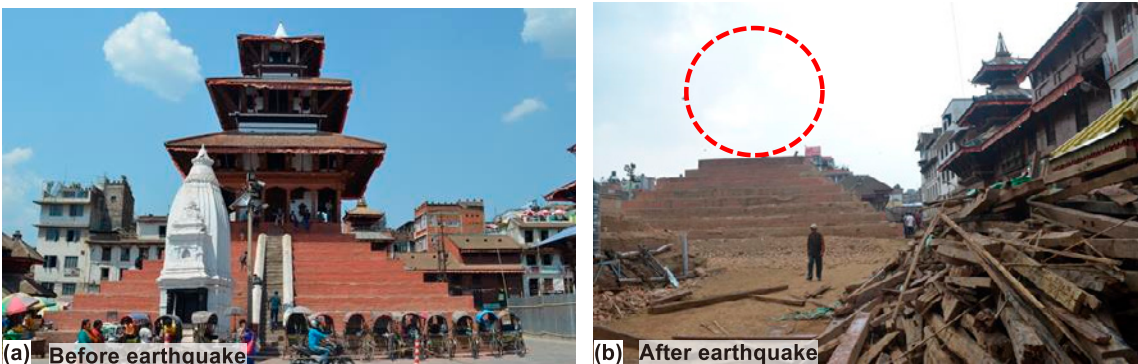
Fig. 13. Maju Deval temple built in 1690 A.D. (a) before the quake (Courtesy: http://hanumandhoka.gov.np/ ) and (b) collapsed all three-stories after the quake.
