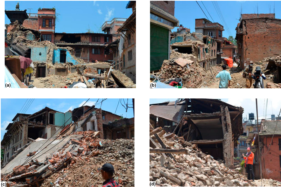
Fig. 6. Entire Newar ethnic town of Bungamati was damaged due to main shock and aftershock. This place is enriched in wooden handicraft business and UNESCO announced the area as the World Heritage sector.
