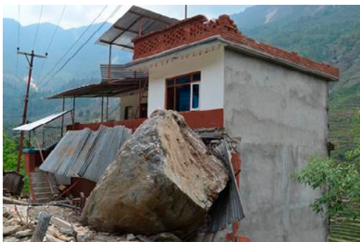
Fig. 26. Intact house shattered by earthquake triggered landslides along the Araniko Highway.
