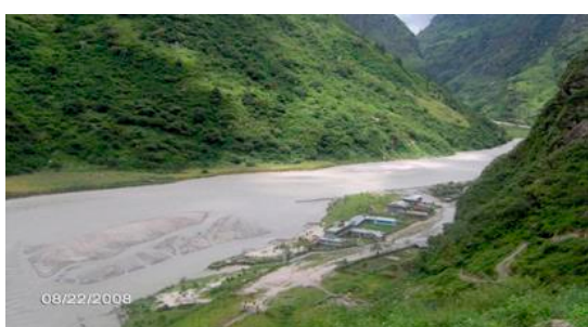
Fig. 9. Landslide dam of Tal Bagar in the Marsyangdi River.
