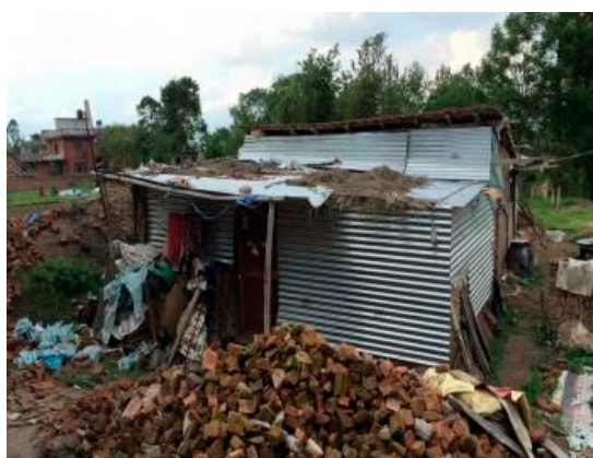
(a) Investigated shelter
