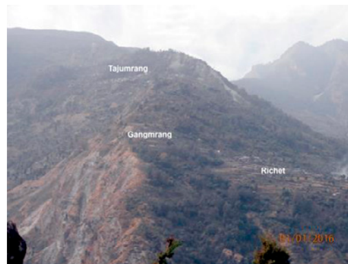
Fig. 16. Some large rock falls and rockslides at Richet and Tajumrang villages. View to W.
