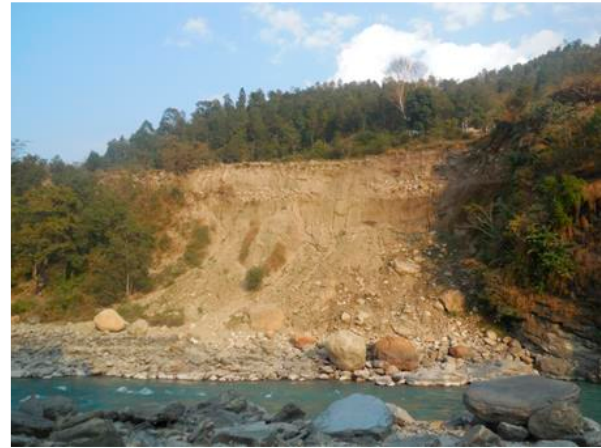
Fig. 4. Landslip on left bank of Budhi Gandaki River at Galane.
