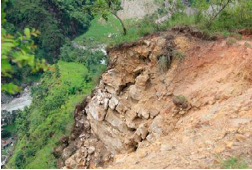
Fig. 30. Open joints in pale yellow to white calcareous quartzite exposed at the crown of the rockslide and rock fall zone lying about 300 m above the riverbed. View to NW.
