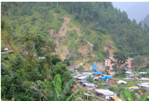
Fig. 34. Rock and debris falls from the south-facing slope of Singati. View to N.
