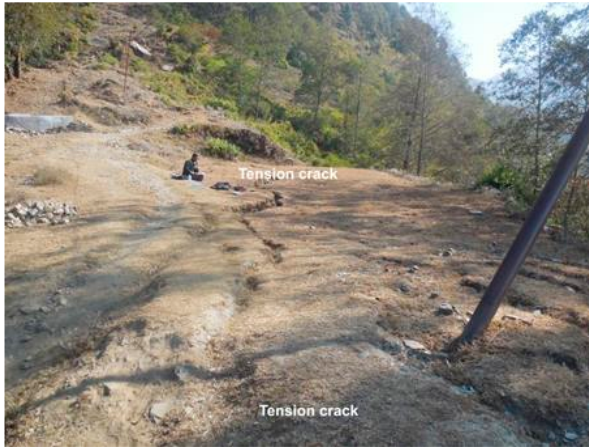
Fig. 3. Tension cracks at about 100 m NE of NTC mobile tower, Barpak. View to W.
