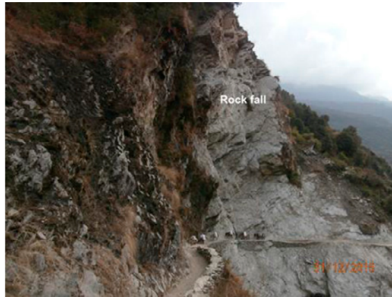
Fig. 14. Rock fall affecting the trail above Gobregau village.
