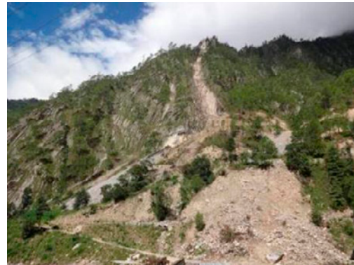
Fig. 20. Rock fall entering the area surrounding the valve chamber and severely damaged road on the talus cone below the portals. View to SW.
