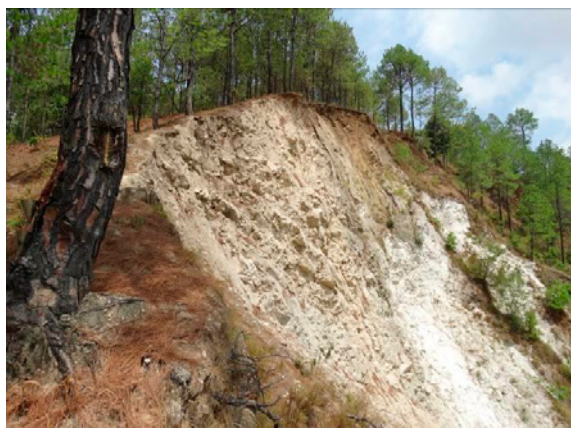
Fig. 36. Reactivated landslide at Pipaldanda. View to NNE.
