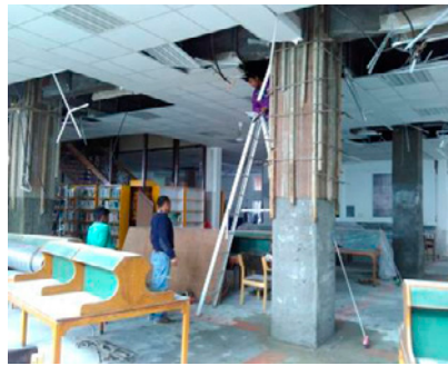
Fig. 15. Concrete jacking of Column, Kathmandu University Central Library, Dhulikhel.
