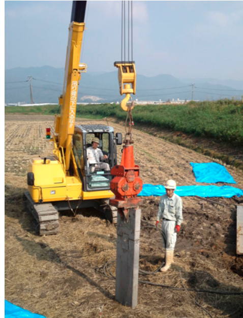
Fig.6 Geotechnical survey using Geoslicer at the retarding basin near No.5 Nokoshi
