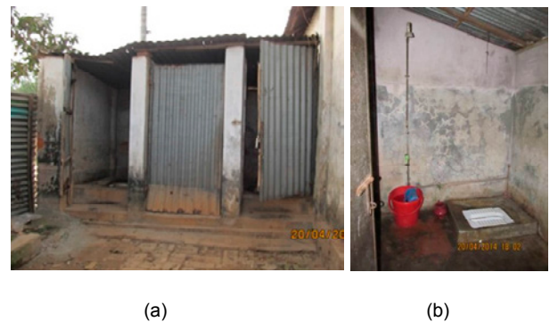
Fig. 16. Example of toilet and bathing facility in workers housing; (a) Shared toilets; (b) A combined toilet and bathing facility.
