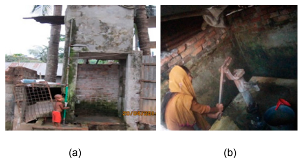
Fig. 18. Water supply facility in the study area (a) Piped water supply with overhead storage tank from deep tube well (b) Hand-operated tube well.
