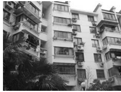
Fig. 7. Current appearance of case building.
