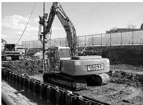
Fig.2 Construction of the MITS method
