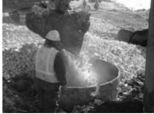
Fig. 3 Placement of rockfill into the drilled shaft
