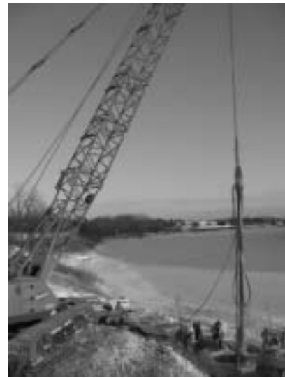
Fig. 4 Compacting rockfill columns with vibrance
