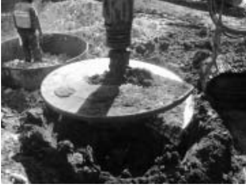
Fig. 2 Drilling for installation of rockfill columns
