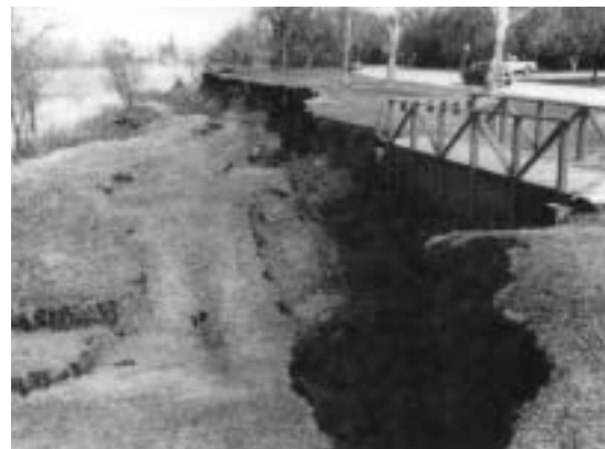
Fig. 1 Instability along riverbanks
