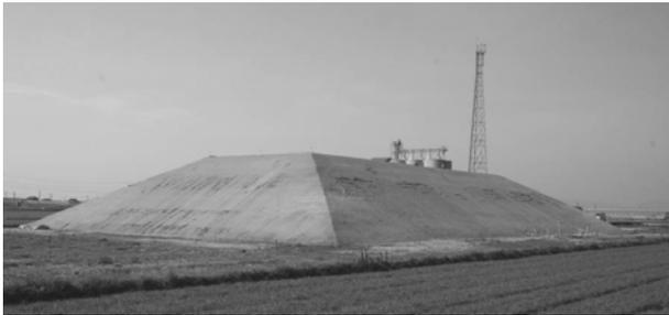
Fig. 6 Completed trial embankment on soil-cement column improved ground
