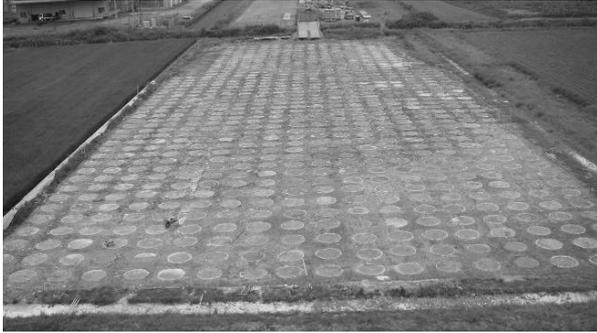
Fig. 5 The state after the soil-cement column improvement
