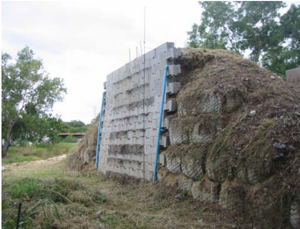
Fig. 9 Completed full scale test embankment construction (Kanjananak 2006)
