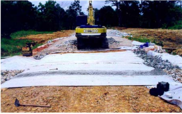
Fig. 4 Completion of prestressing work on geosynthetic reinforcement (after Chew et al. 2005)
