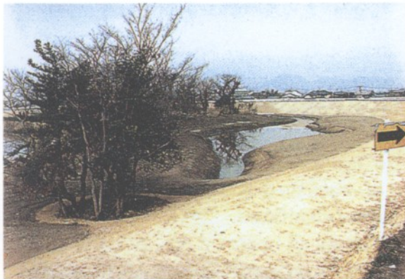
(a) Just after river works
