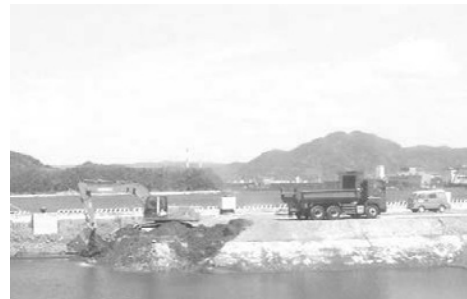
Photo 9 Backfilling by backhoe
