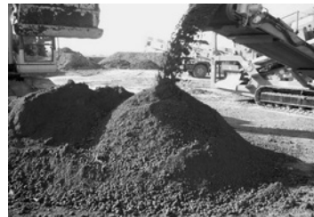
Photo 13 Improved embankment soil
