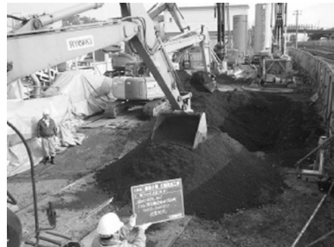
Photo 27 Backfilling of the insolubilized soil
