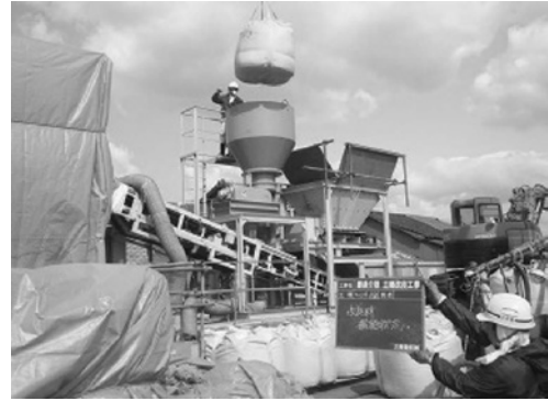
Photo 25 Insolubilizing agent was added
