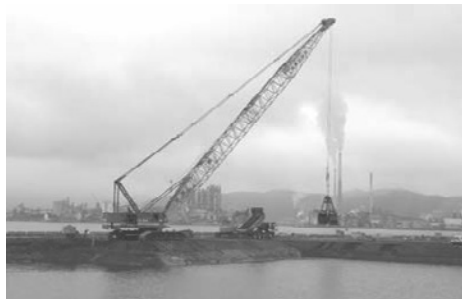
Photo 8 Backfilling by clamshell
