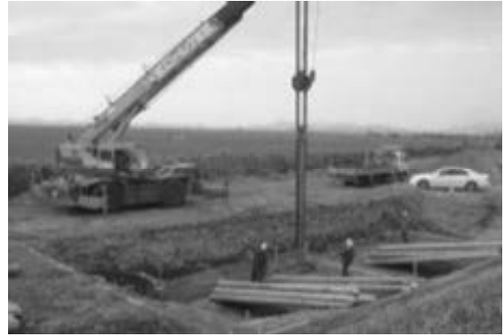
(b) Installation of wooden piles
