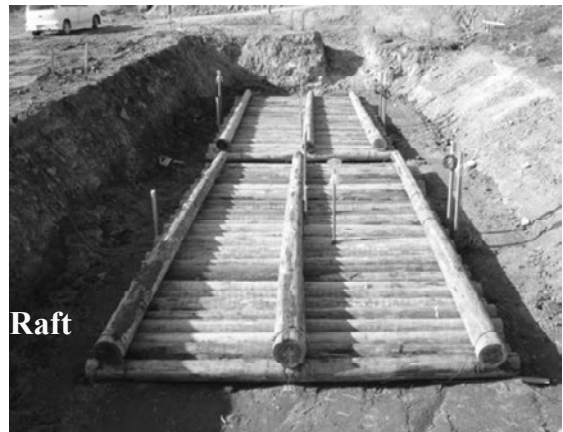
(d) Constructions of two sets of wooden rafts
