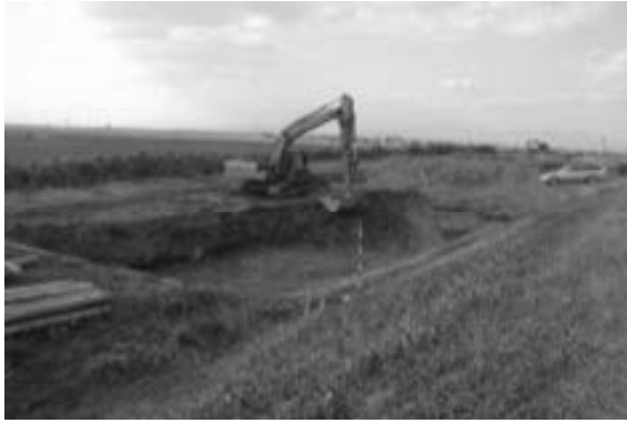
(a) Excavating to meet groundwater level
