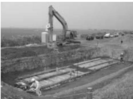
(e) Under backfilling
