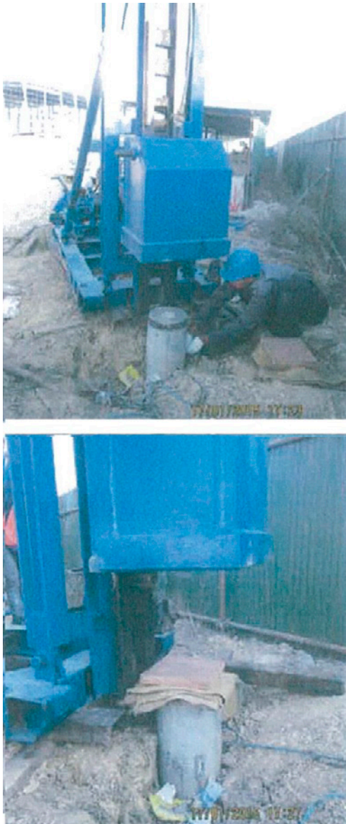
Fig. 13. The dynamic pile load test on micro spun pile.
