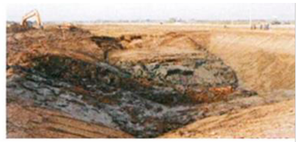
Fig. 2. Trial excavation work.
