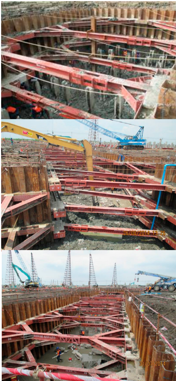
Fig. 4. Sheet pile braced excavation system.
