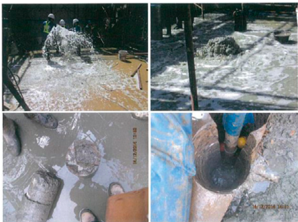
Fig. 7. Concrete coring at location 1.
