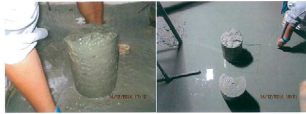
Fig. 8 . Concrete coring at location 2.
