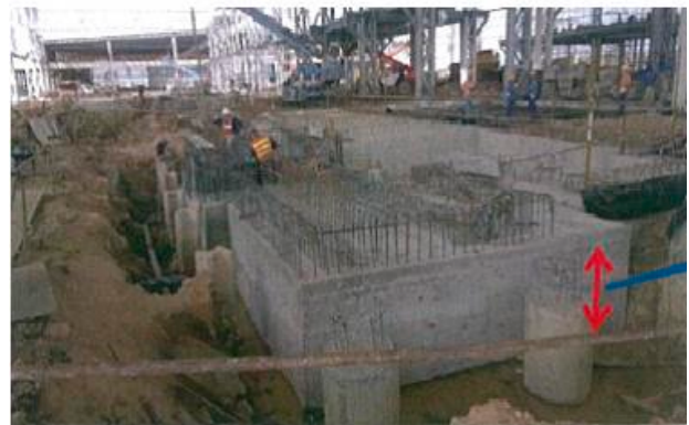
Fig. 12. The piling work of micro spun pile.
