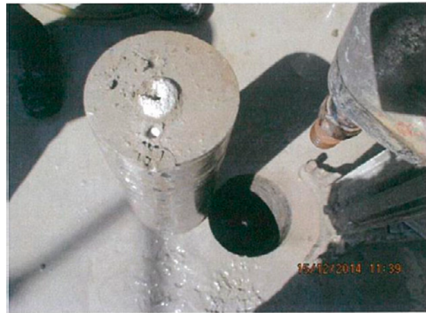
Fig. 9. Concrete coring at location 3.
