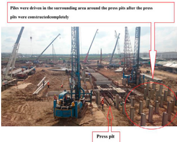
Fig. 6. Piles driven in the surrounding area of the press pit.
