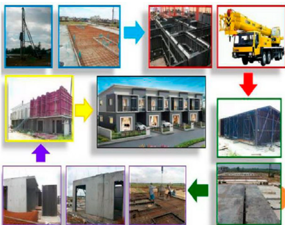
Fig. 6. 2-story-Townhouse Building in the process.
