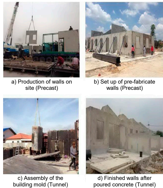
Fig. 1. On-site Application of LMP.
