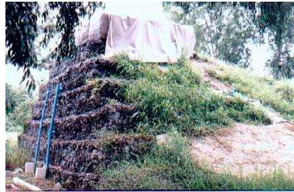
Fig. 16. Completed hexagonal wire mesh reinforced embankment (Teerawattanasuk, 2004).
