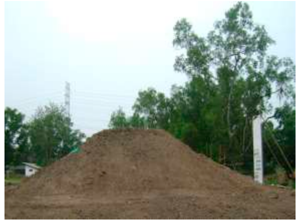
Fig. 5. Completed LLGs reinforced embankment construction.
