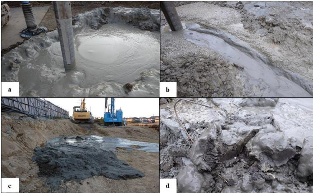
Fig.1: Non-solidification in the implementation of DMM on a construction site.
