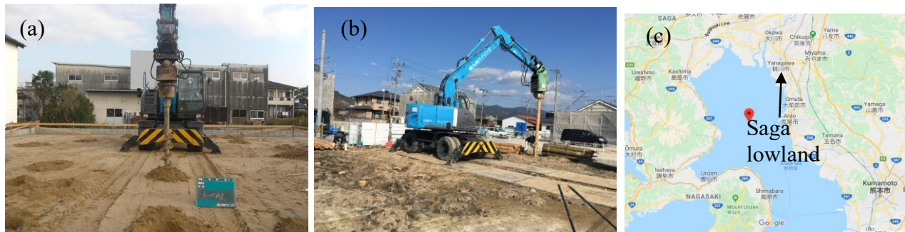
Fig. 1. (a) Auger drilling, (b) Installation of timber pile, (c) Saga lowland
