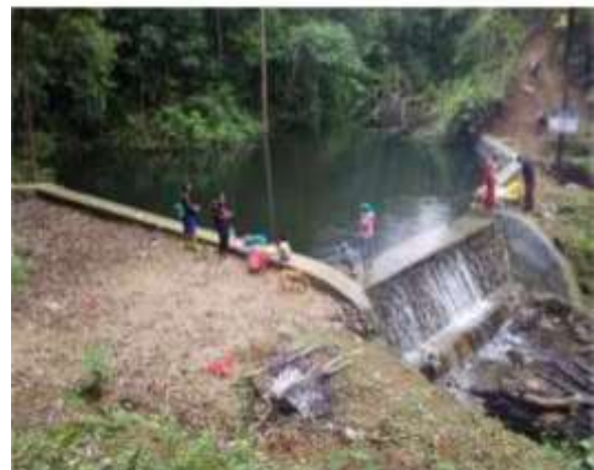
Figure 2. The Embung construction in patinro Village
