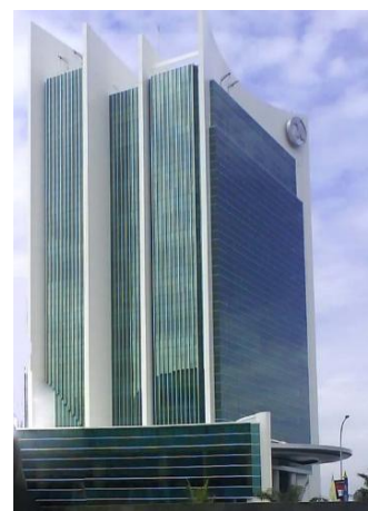
Figure 2. Mega Bank Makassar Tower Building
