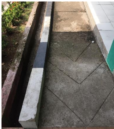
Figure 7. Ramp beside hostel
