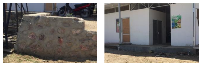
Figure 16. The liquid waste disposal pipe
