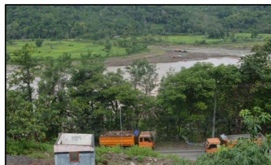
Figure 1. Erosion on the Jeneberang River due to mining activities
