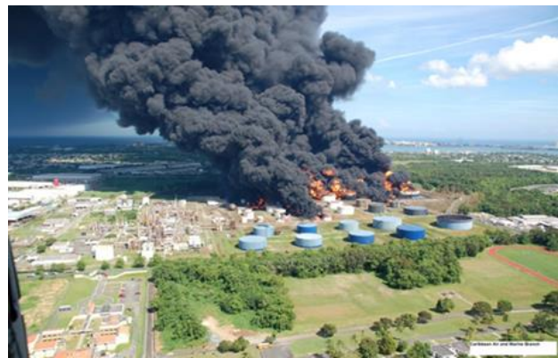
Figure 11. Massive fire in CAPECO tank terminal [5]
