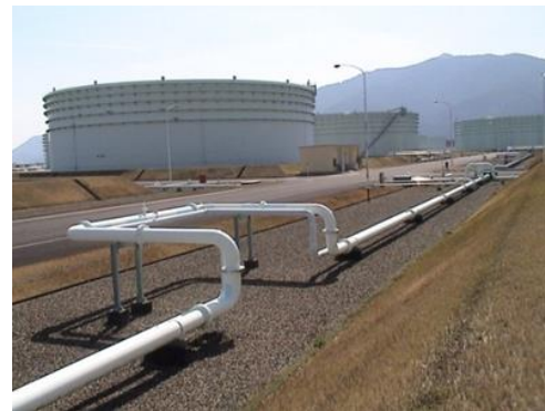
Figure 1. Aboveground storage tank (AST)
