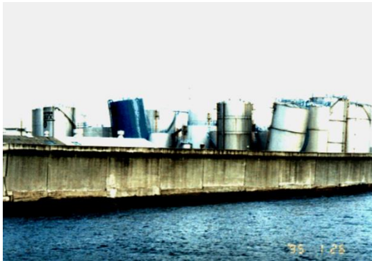
Figure 12. Inclination of small ASTs due to the soil liquefaction in Kobe at the 1995 Kobe Earthquake (Courtesy of National Research Institute of Fire and Disaster, Japan)
