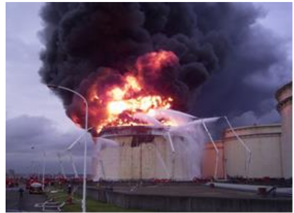
Figure 13. Full surface fire in a 30,000m 3 naphtha storage tank in Tomakomai at the 2003 Hokkaido Earthquake (Courtesy of National Research Institute of Fire and Disaster, Japan)
