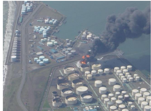
Figure 14. Aerial photo of full surface fire in a 30,000m 3 naphtha storage tank in Tomakomai at the 2003 Hokkaido Earthquake (Courtesy of National Research Institute of Fire and Disaster, Japan)
