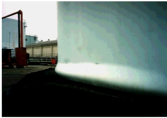
Figure 11. Elephant foot bulge of a sidewall in a small AST in Kobe at the 1995 Kobe Earthquake (Courtesy of National Research Institute of Fire and Disaster, Japan)
