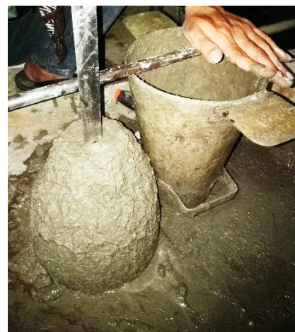
Figure 4. Concrete slump testing
