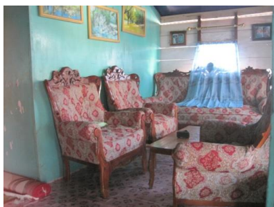
Figure 9. Living room is rarely functioned and filled with furniture that is quite heavy and disproportionate with the space so that it affects the construction of floors (planks) which are sag.
