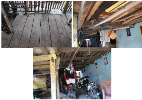
Figure 15. Materials in floor and basement
