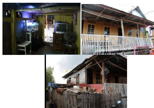
Figure 14. Materials in the wall
