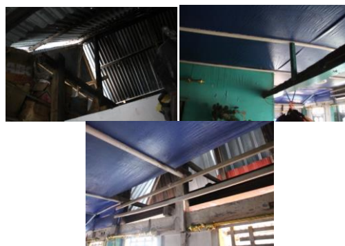
Figure 13 Materials in the roof
