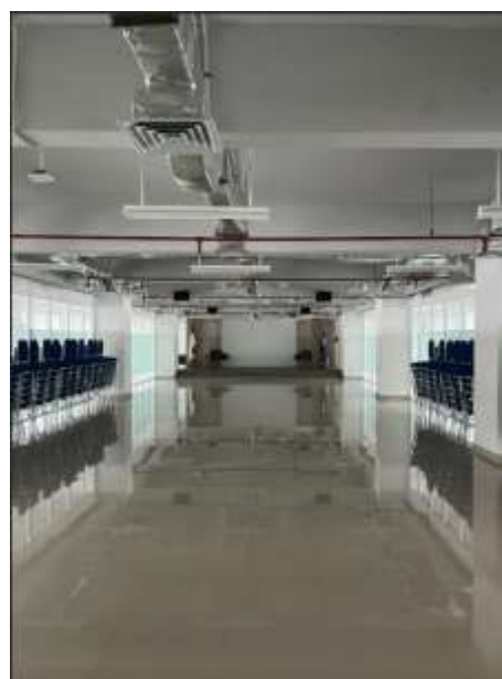
Figure 4. Interior condition of student lounge
