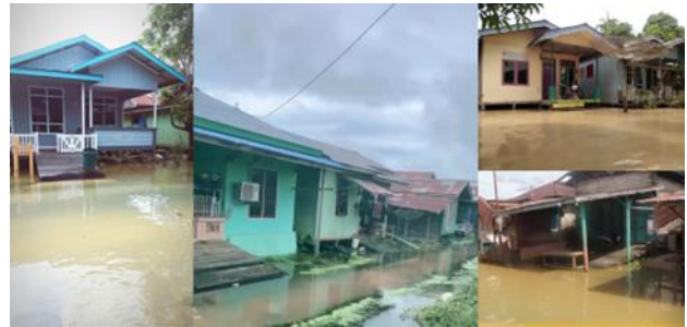
Figure 6. Flooding on the stilt house
