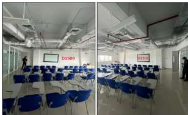
Figure 7. Interior Condition of Classrooms D1509 and D1510
