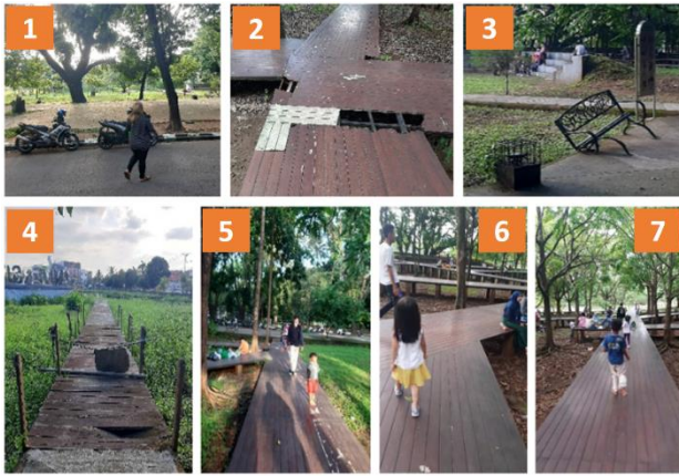
Figure 21. Cautiousness behavior of visitors about park facilities: 1. Visitors cross to the park from the parking location; 2. Condition of a damaged pedestrian in the wetland area; 3. Broken bench; 4. The condition of the wooden bridge towards the infinite bridge pier; 5,6,7. Adult visitors and children in the wetland area
