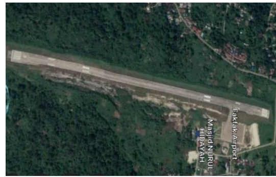
Figure 2. General view from the Torea Fakfak airport
