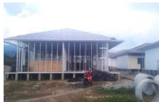
Figure 5. Mild steel structure in Petobo shelter
