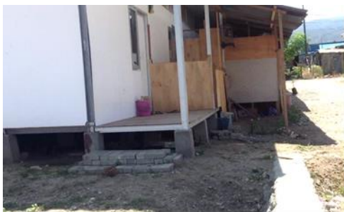
Figure 27. Stairs to help ascend to the residential units
