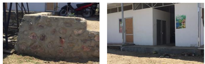
Figure 16. The liquid waste disposal pipe
