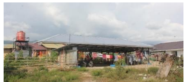
Figure 15. Solar cell in shelter of Petobo
