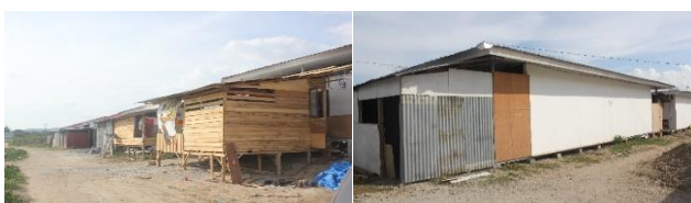
Figure 18. The addition of space in the units of Petobo shelter
